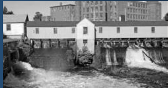
Mill dams in Lowell, MA on the Merrimack River
